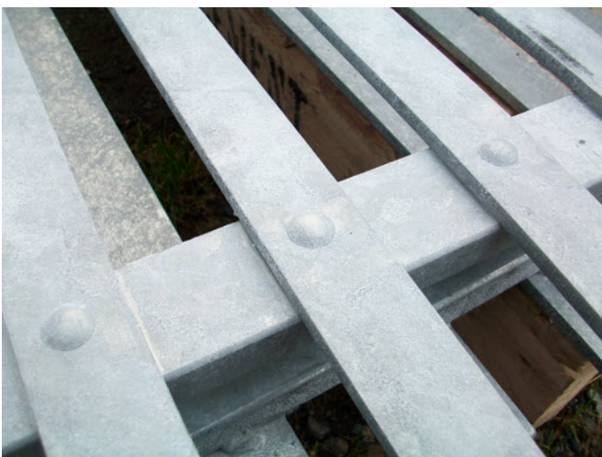
Photograph 5. Close up view of the simulated rivets on a finished gate.
